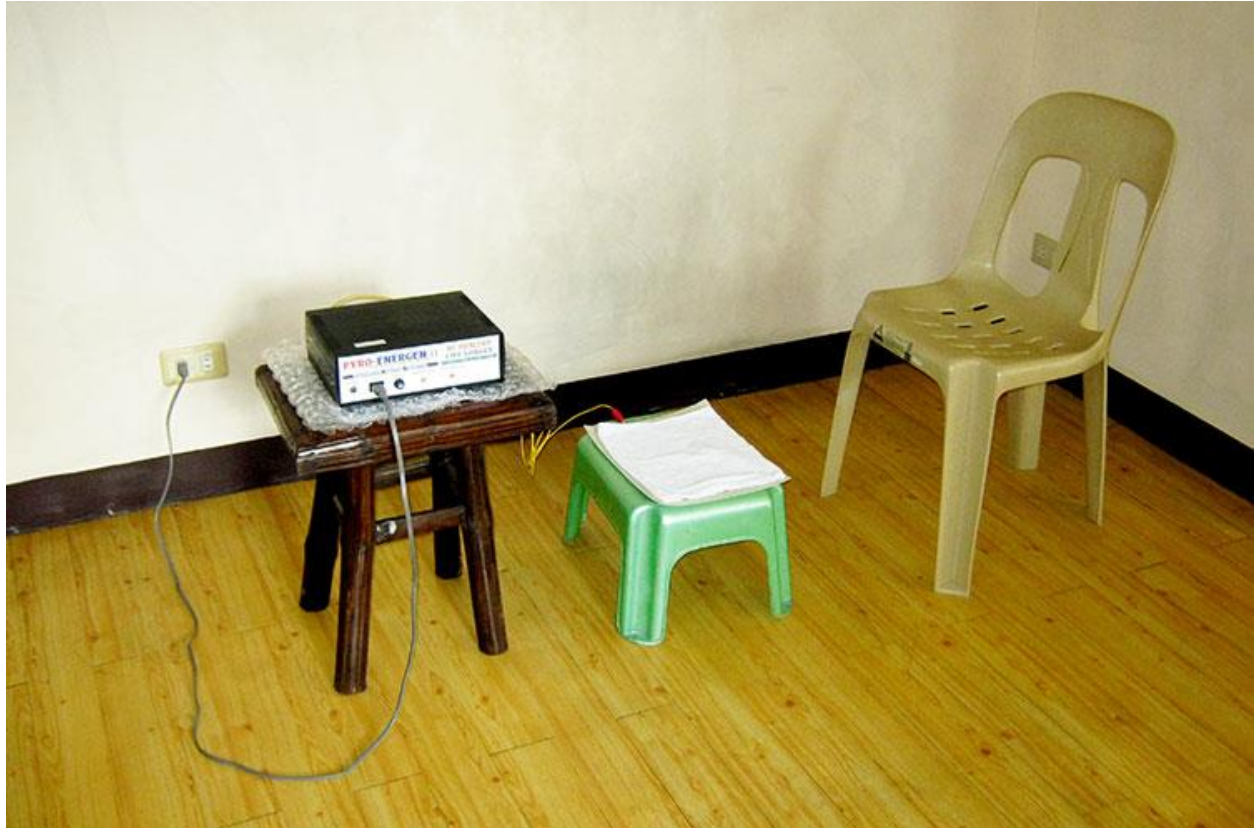
Sample PYRO-ENERGEN machine Installation – Therapy Area
